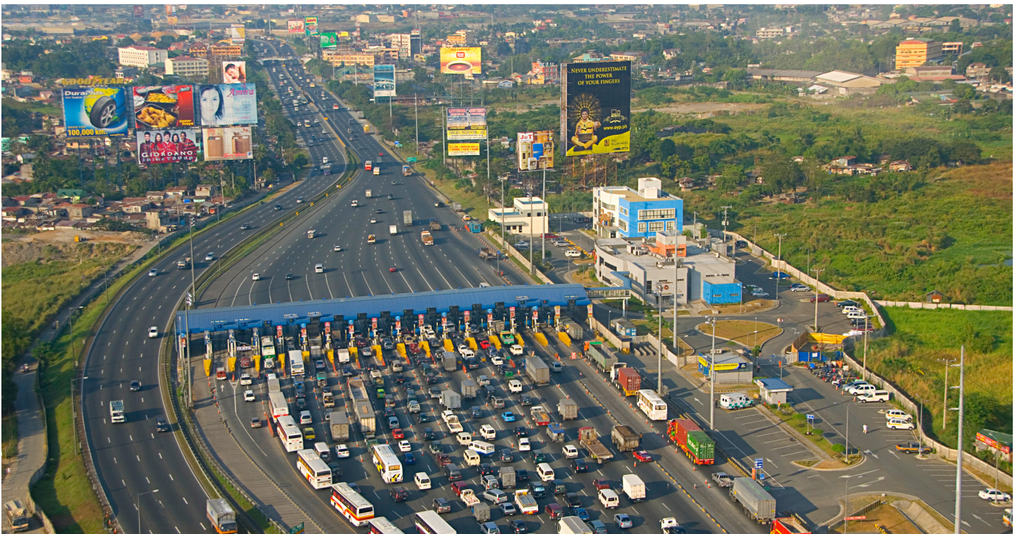
The ADB-supported North Luzon Expressway Rehabilitation and Expansion renovated an 83.7-kilometer section of road from Manila to the Clark Special Economic Zone in Pampanga province by building or rehabilitating 14 interchanges, 24 bridges, and 31 overpasses. The road used to be a heavily pot-holed two-lane thoroughfare, where trucks, buses, and private vehicles dangerously competed for space. Today, it is a safe, smooth tollway with good lighting, modern signage, and vigorously enforced traffic laws. Photo by Kevin Hamdorf. ADB Photo Library.
